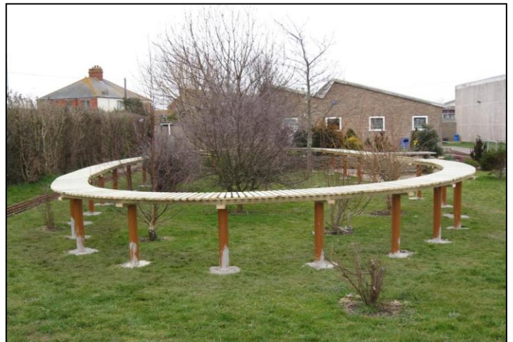
The completed oval
