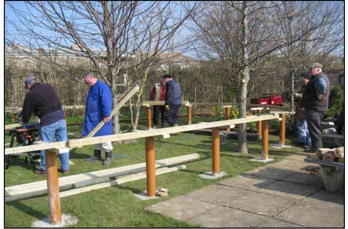
Team work as the structure is built
